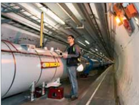
Nedo products in use at CERN
