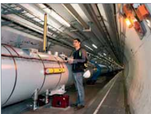
Nedo products in use at CERN
