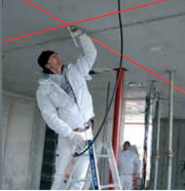
Simple transposition of plumb points and lines onto the ceiling.
